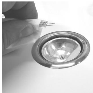
Step 5. Using a tissue or gloves to protect bulb, fit new halogen bulb. (Oil from the skin can affect halogen bulbs)
