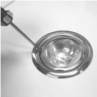
Step 1. Remove lamp cover using a small screwdriver, there are 4 points to assist in easy removal
