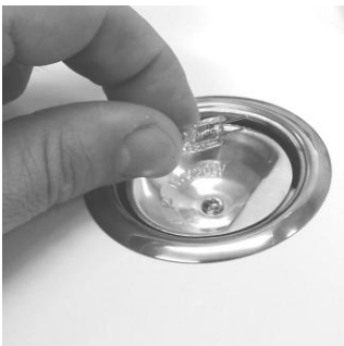
Step 4. Remove lamp and discard in a safe and proper manner.
